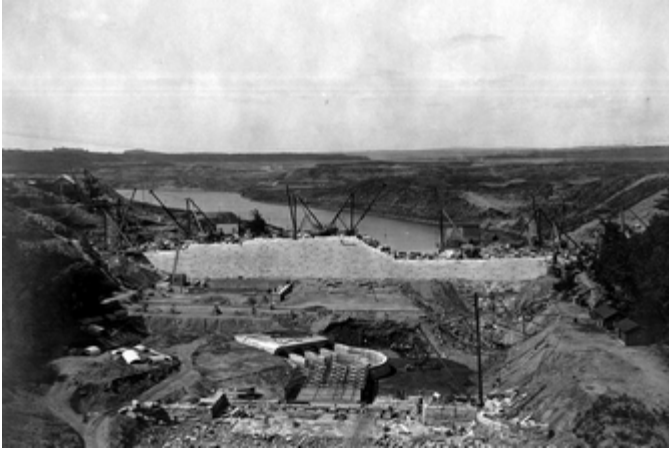
Construction of the dam.
